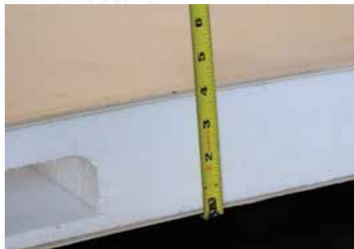
4" thick roof with built-in insulated A/C ducts.
