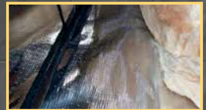
Radiant shield Thermo-foil – R-38.
