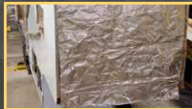
Radiant shield Thermo-foil – R-38.
