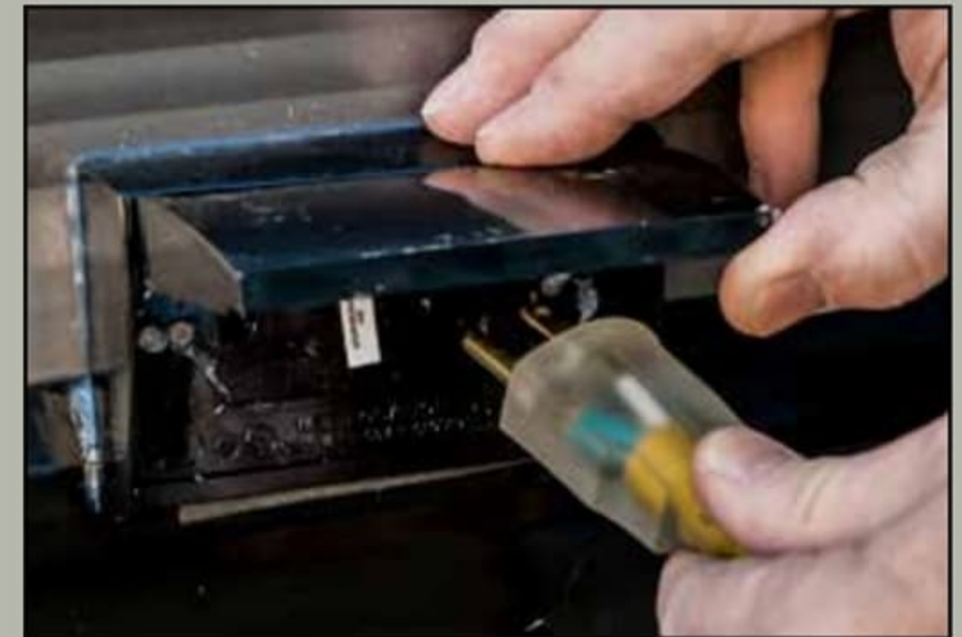
Convenient Outside GFCI Protected and Covered Outlet.
