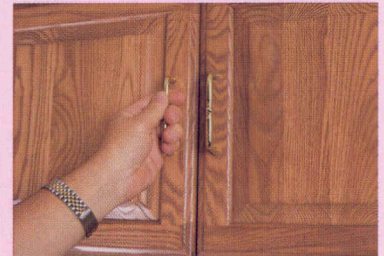
These wider door handles make it easier to open and close cabinet doors and drawers.
