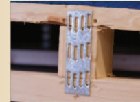
US Vertical wood studs for added support.
