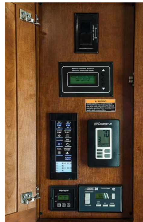
Important gauges, switches, and controls are all centrally located in the OnePlace® Systems Center .
