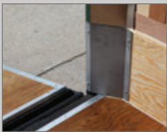
GALVANIZED STEEL PLATE PROTECTS CORNER POST
