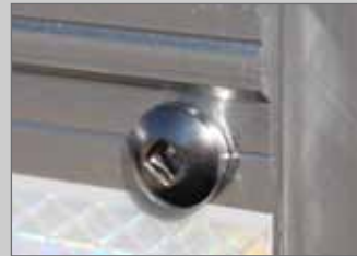
EXTERIOR SCREWS ARE STAINLESS STEEL
