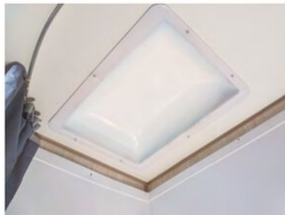
Skylight over Shower
