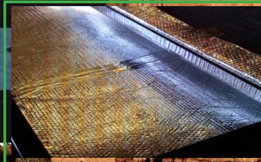
Reflective Insulation Blanket Applied to Roof, Slide-Out Floor, Entire Underbelly, Additional Wrap Around Holding Tanks
