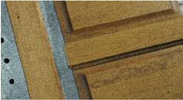
Raised panel door detail
